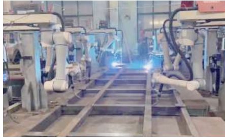
Steel Frame Welding
